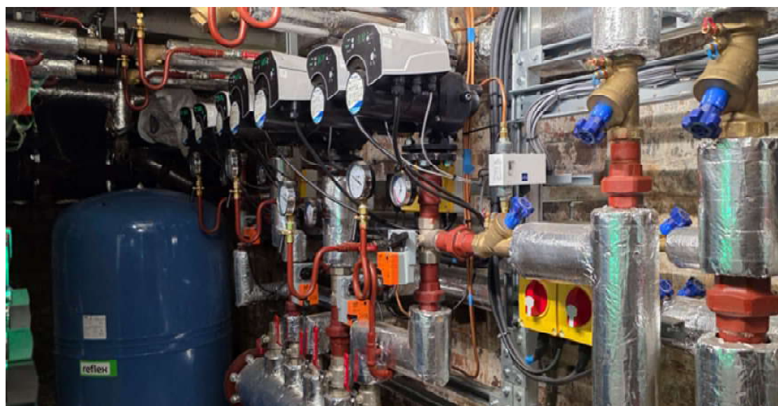
Photo showing new plant following replacement of school heating system
